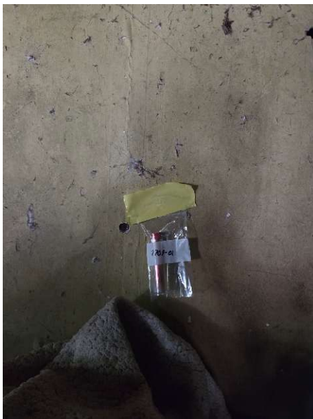
Sample 2709-01 Typical Drywall & Joint Compound
